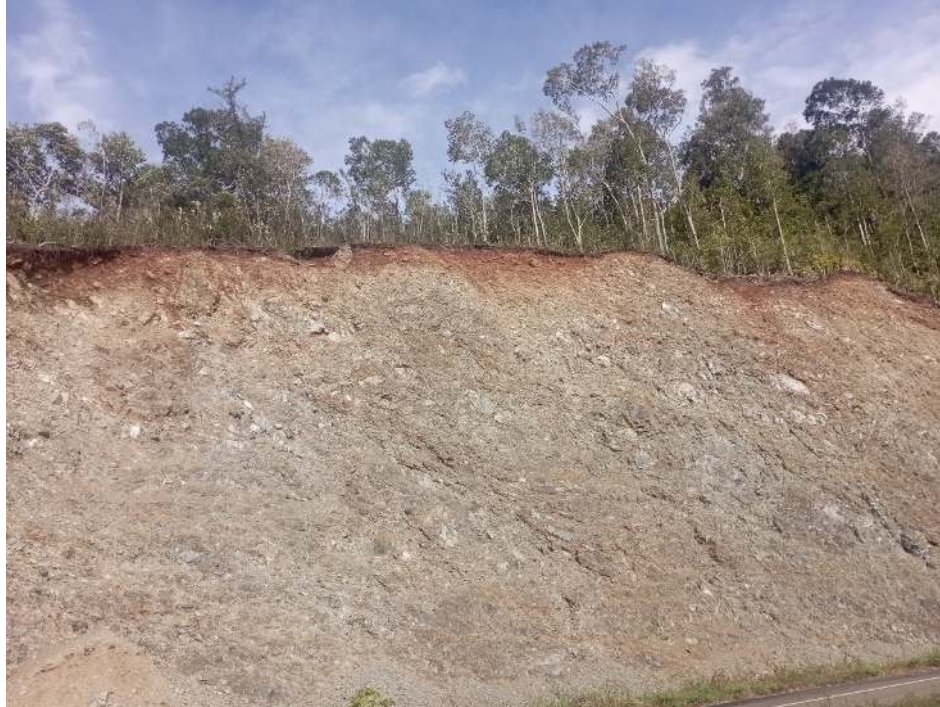
Figure 1 Field photograph of the investigated road-cut slope exposing highly weathered serpentinite mélange characterized by extensive fracturing, heterogeneous rock mass, and steep excavation geometry.
